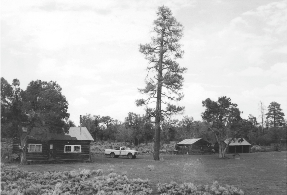
Figure 1. Horse Valley Ranch, 1966. View looking north-northeast. From left to right: the ranch house, the original cabin (in use as a feed shed), and the barn. From Patrick D. Nolan, An Appraisal of the J.D. Waring Ranch located approximately 95 miles south of St. George, Utah , 1966, Waring land files (L1425), Lake Mead National Recreation Area headquarters, Boulder City, Nevada.
