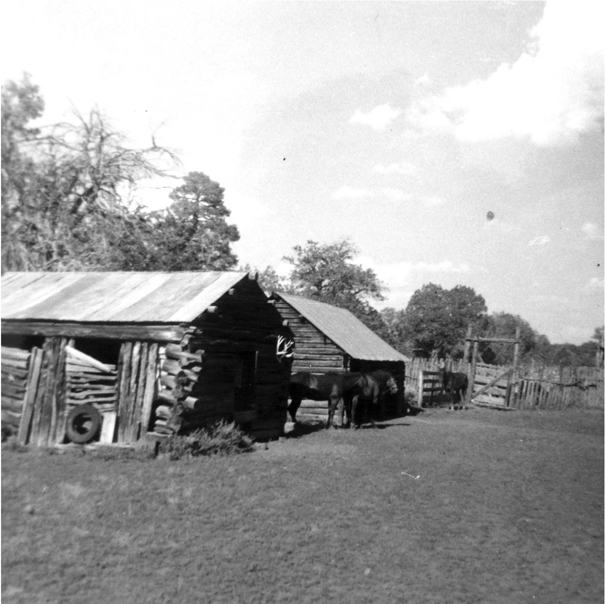
Figure 5. The original cabin (in use as a feed shed), the barn, and the corrals, Horse Valley, 1966. View looking east. From Western Farm Management Company, Appraisal Report of Waring Ranch, Mohave County, Arizona, for National Park Service , [1966], Waring land files (L1425), Lake Mead National Recreation Area headquarters, Boulder City, Nevada.
