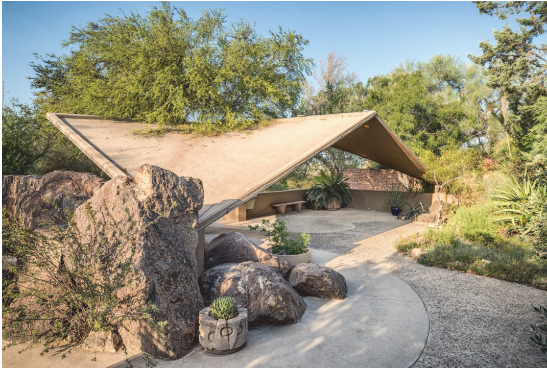
Figure 2. Entrance to Sunset Garden, facing southwest (Jude Ignacio and Gerardine Vargas, June 2015)
