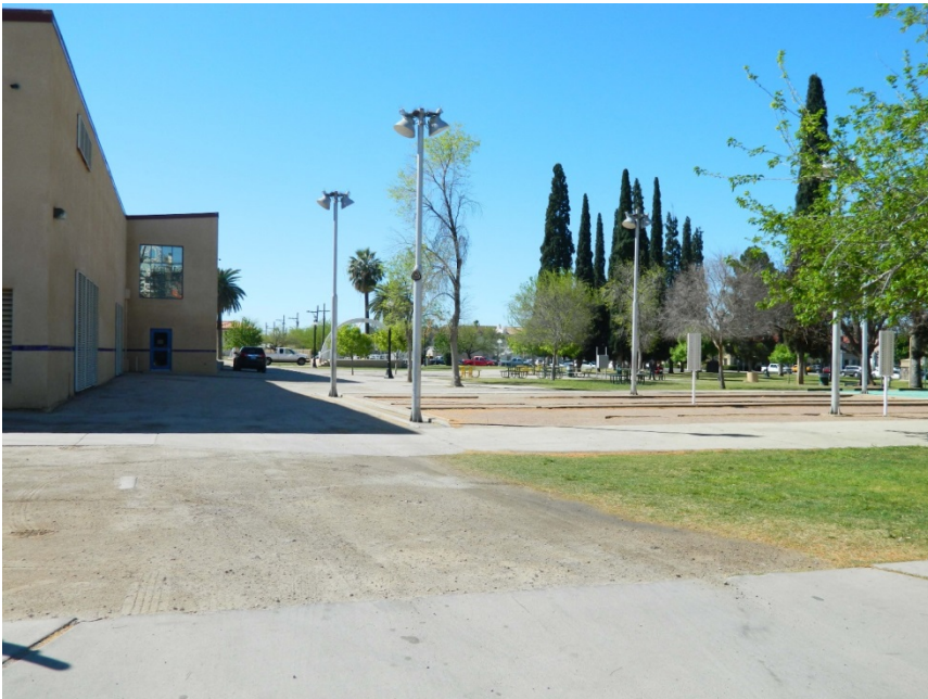
Figure 2. Maintenance driveway behind Armory Park Center. View looking south towards 13th St. Stephanie Badurski, 2017.
