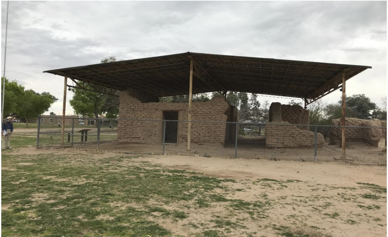
Figure 1: Original adobe hospital, facing west. (Fermin Garcia, 3/24/18)
