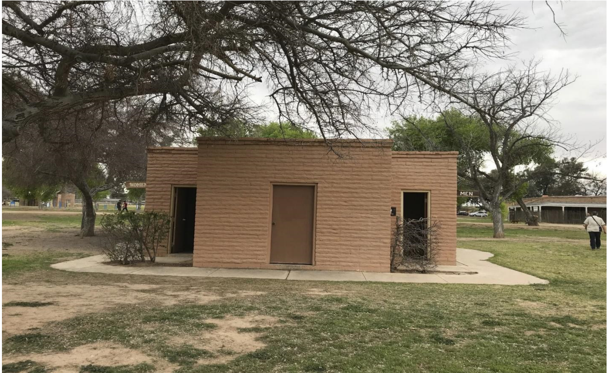
Figure 3: Newer restrooms, facing south. (Fermin Garcia, 3/24/18)
