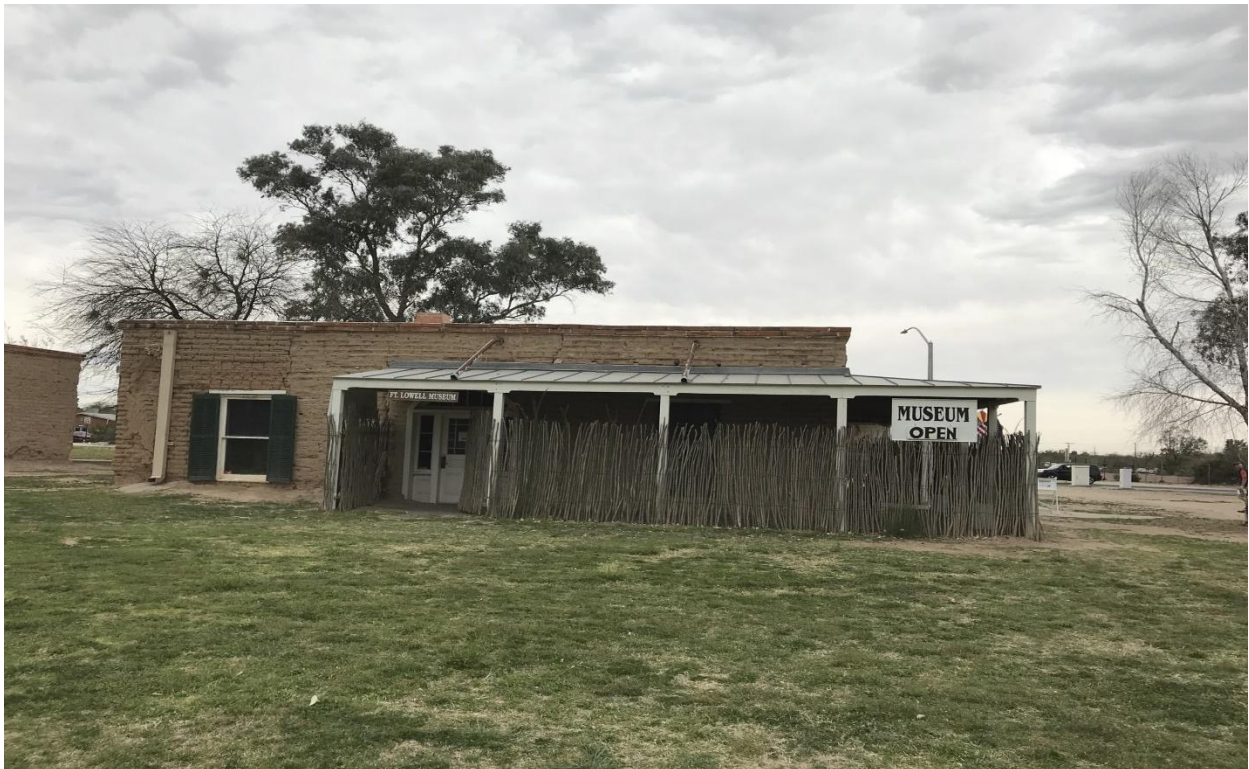
Figure 2: Fort Lowell History Museum, facing west. (Fermin Garcia, 3/24/18)
