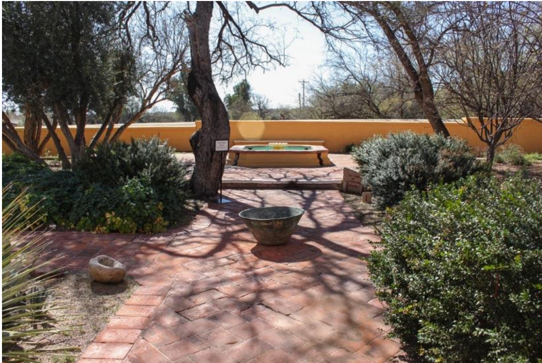
Figure 21: Visitor Center garden fountain with view of brick paths laid by CCC workers, facing south (Starr Herr-Cardillo, February 2014).
