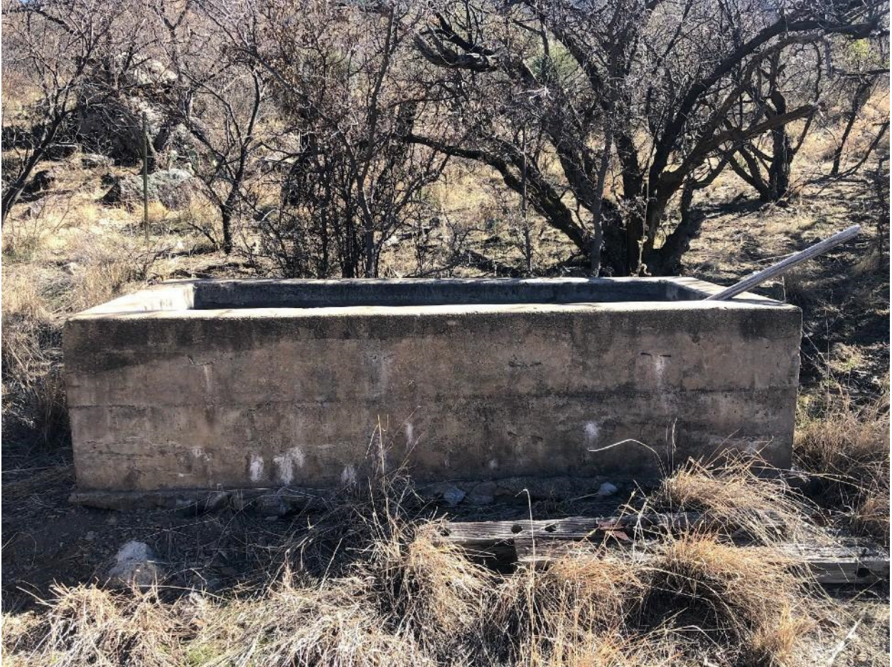
FIGURE 5 - Concrete water trough facing southeast, photo by Melanie Olson, 02/06/21.
