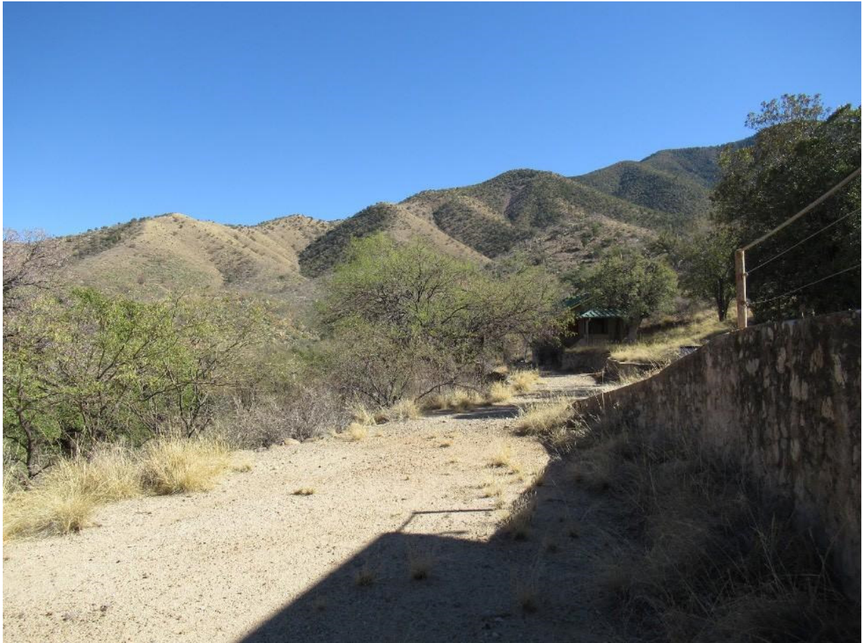
FIGURE 2 - View shed and retaining wall below USBS Cottage (C25) facing southeast, photo by Sarah McDowell, 02/06/21.
