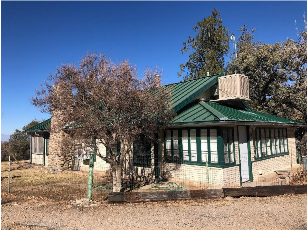
FIGURE 6 - Caretaker's house (C-9) facing northeast, photo by Melanie Olson, 02/06/21.
