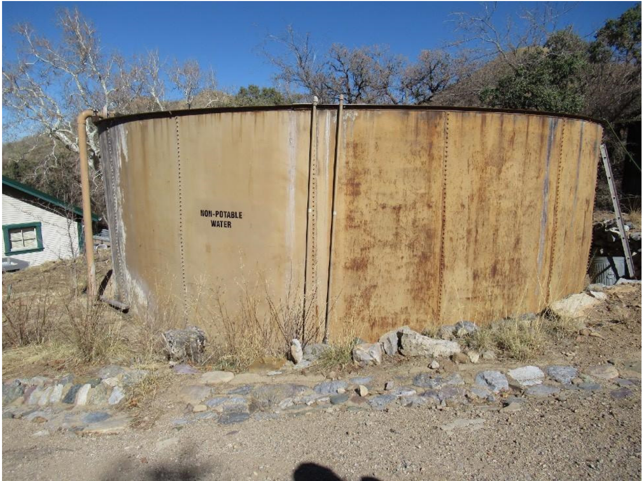
FIGURE 8 - “Non-potable water” tank, and masonry rain drainage feature, facing northwest, photo by Sarah McDowell, 02/06/21.
