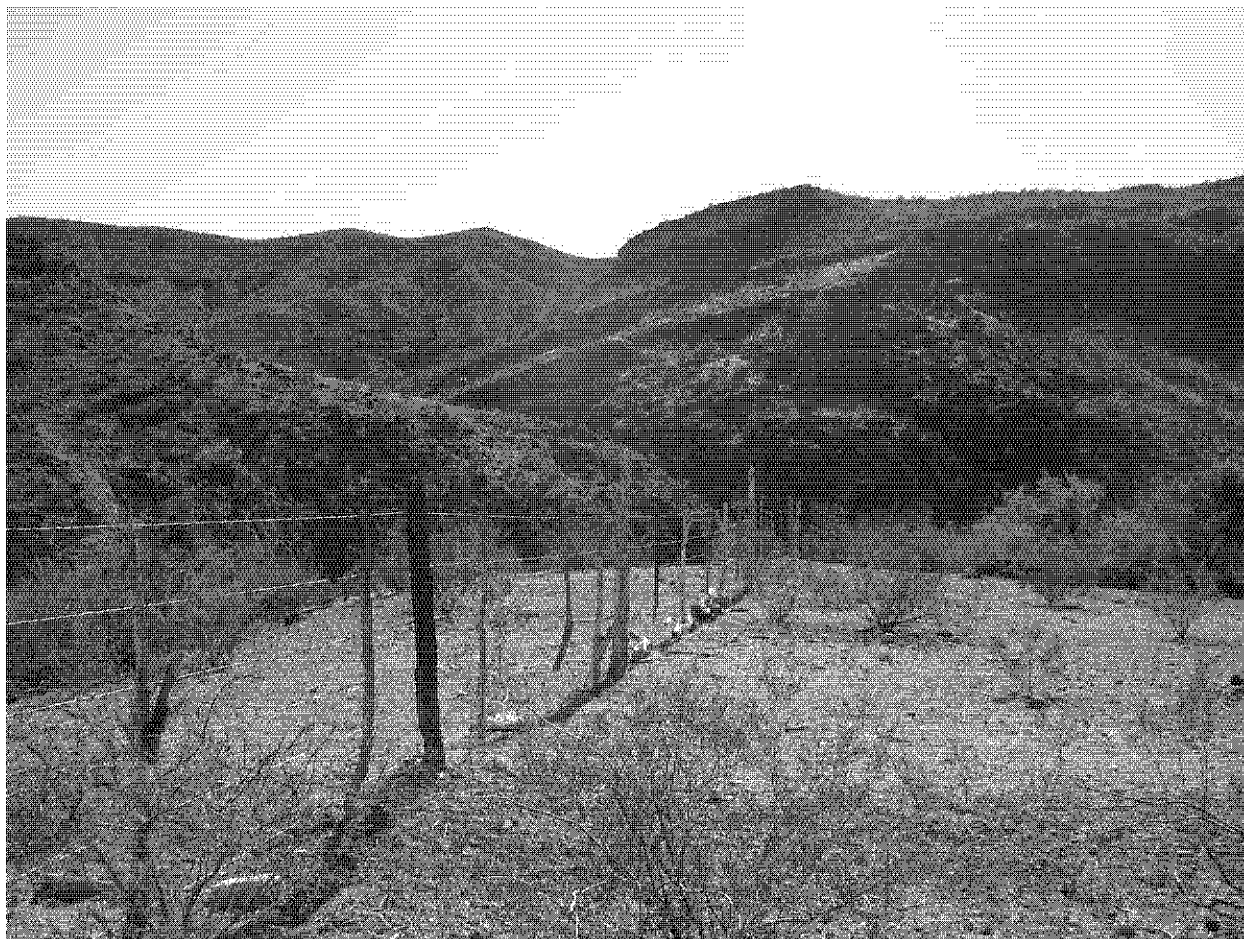
Fig. 12. The restored fence enclosing the pasture above the ranch core, showing the rough wood posts fashioned from native tree trunks and limbs that historically supported most of the barbed-wire fencing at the ranch. Photograph by Alexander Matsov, November 2009.
