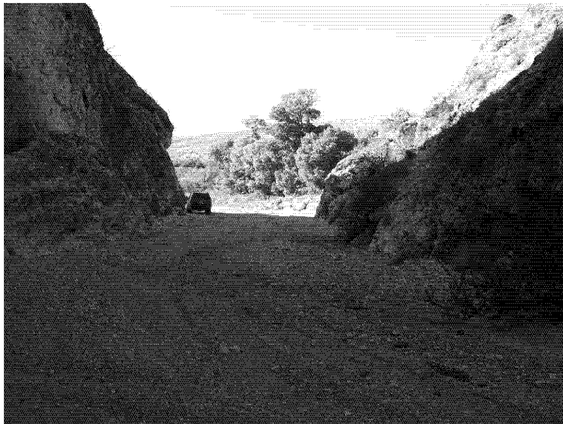
Fig. 2. The narrow walls of this pass, called the Box, tend to channel seasonal flood waters toward the ranch core. Flood damage in 2000 led the National Park Service to install the boulders visible on the far edge of Pigeon Wash as an erosion deterrent. Photograph by Christopher Stevens, November 2009.
