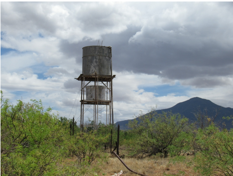
Figure 9: Water tower (McDowell, 2021).
