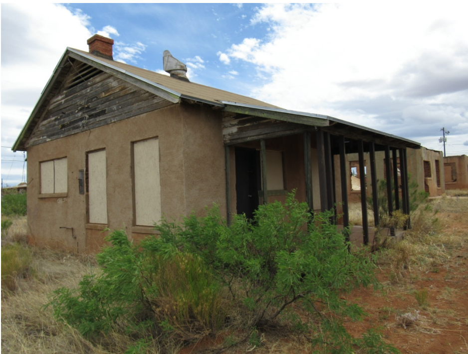
Figure 7: Non-commissioned officers' residence (McDowell, 2021).
