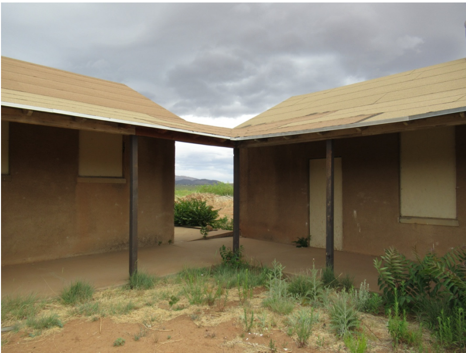
Figure 5: Western quadrangle roof connection between barracks and mess hall (McDowell, 2021).
