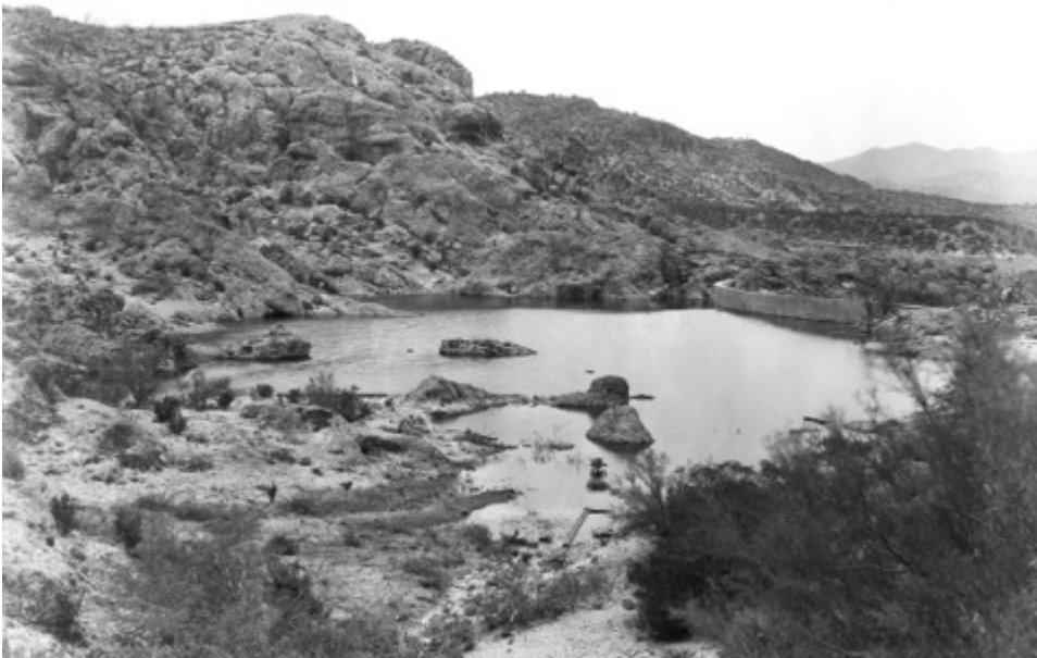
Reservoir 1925, looking west (Courtesy of Boyce Thompson Southwestern Arboretum Archives).
