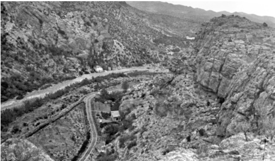
View of the Pumphouse, probably shortly after 1925, looking southwest (Courtesy of Boyce Thompson Southwestern Arboretum Archives).
